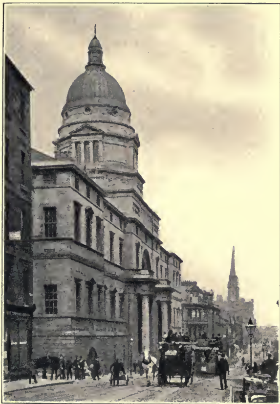
THE UNIVERSITY, SOUTH BRIDGE.
